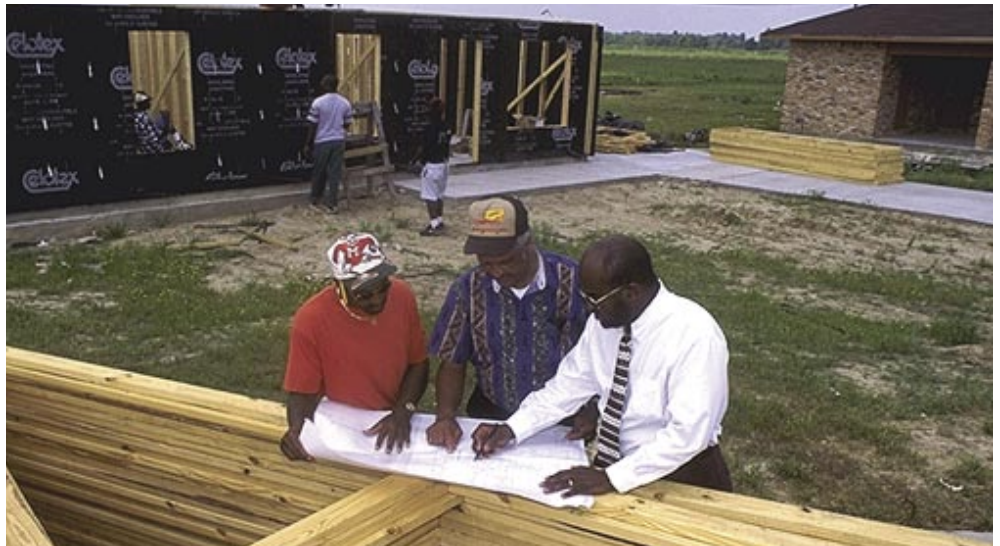
L to R: Daniel Kent, construction foreman, Robert Kent, housing director, and Community Development Manager Sylvester Pomerlee inspect plans for homes in Indianola, MS being built under USDA's self-help program.
